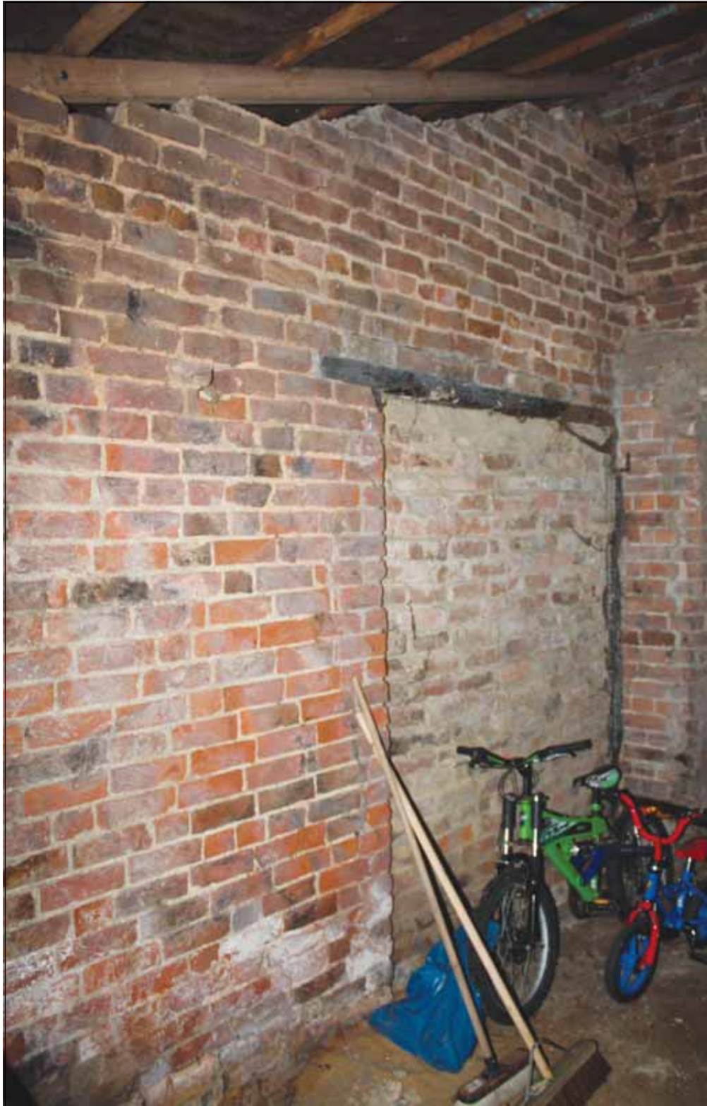
Plate 37: Detail of blocked doorway inside tack room
