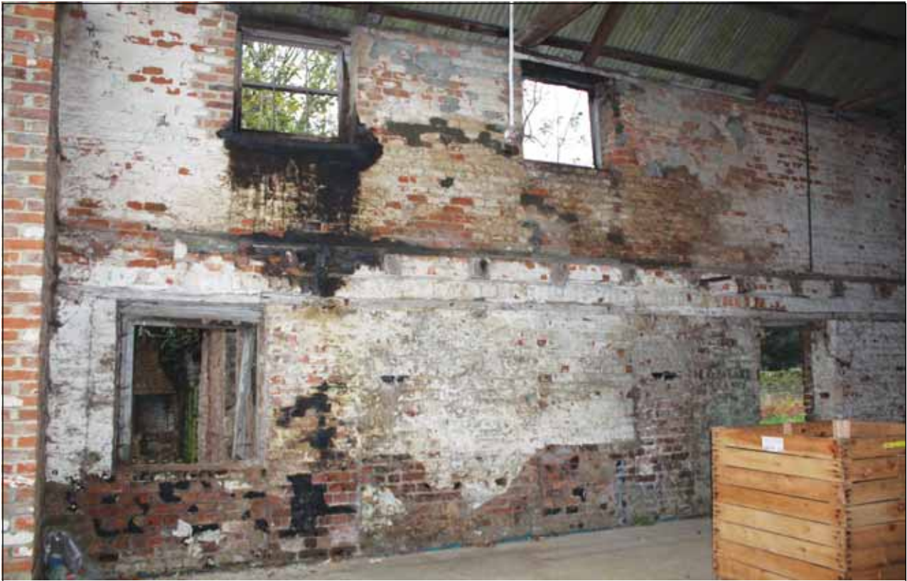
Plate 26: Detail of internal wall showing blocked-up openings, Barn 1
