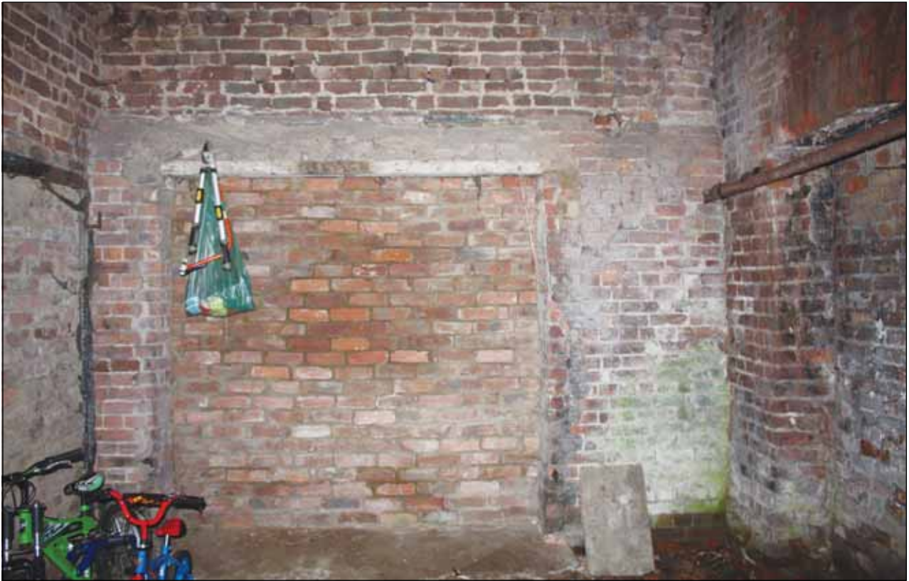
Plate 38: Detail of blocked opening inside tack room
